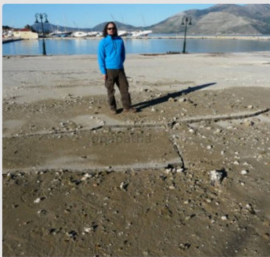
Figure 8. Ejected material in the quay of Lixouri (photo taken on 7/02/2014)
